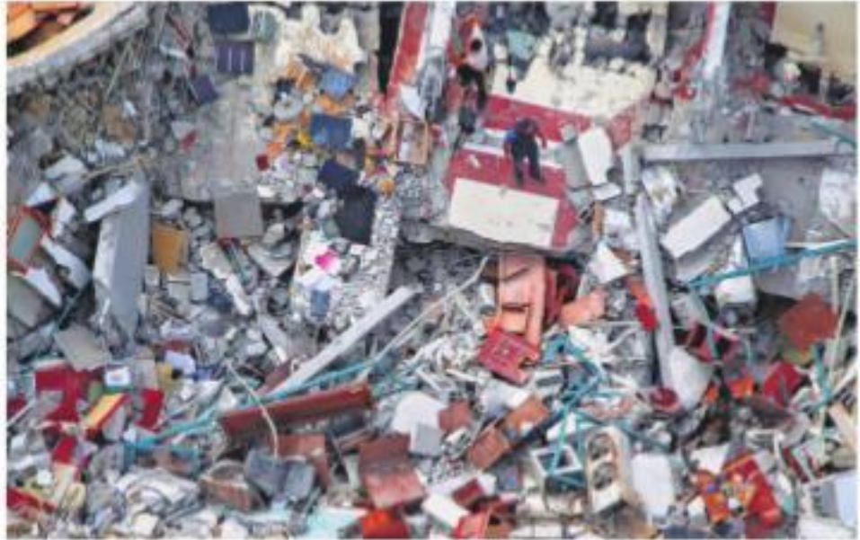
Palestinians on Friday inspect the destroyed building in Gaza City that housed offices of AP and other media, after it was hit last week by Israeli airstrike | AP/PTI
